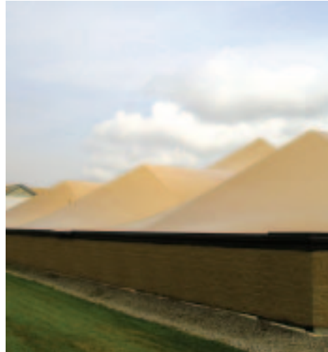
Complex roof lines presented a roofing challenge.
