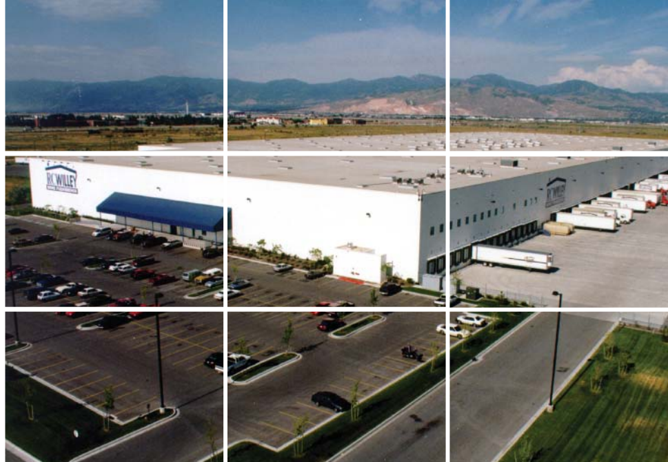
The RC Willey Intermountain Distribution Center in Salt Lake City, Utah utilizing the Sarnafil membrane.
