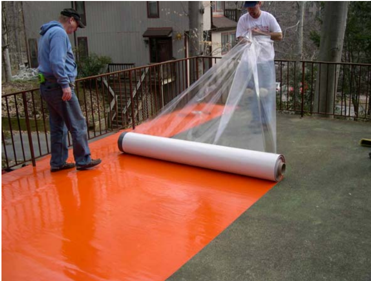
Installation of G476 Self Adhered Membrane on a concrete deck
